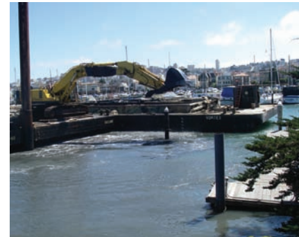
Summer 2010 Maintenance Dredging
